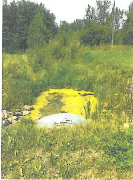
CULVERT C518 DOWNSTREAM END
